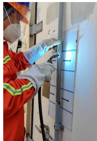
After proper alignment, tack weld.
