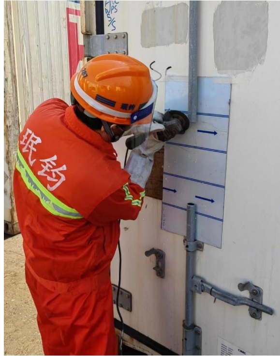
Beveling edges for good weld penetration.
