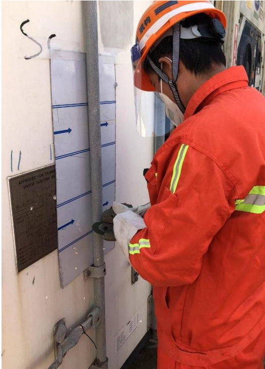
Shielded door panel / cutting disc being used.
