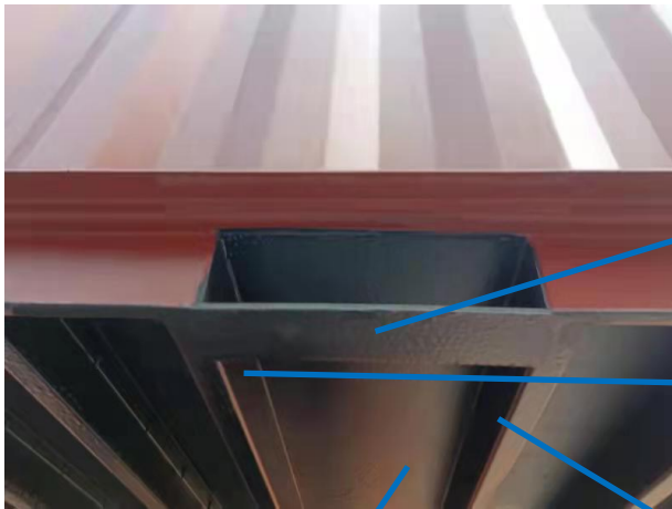
Forklift Pocket Top Plate FLP
