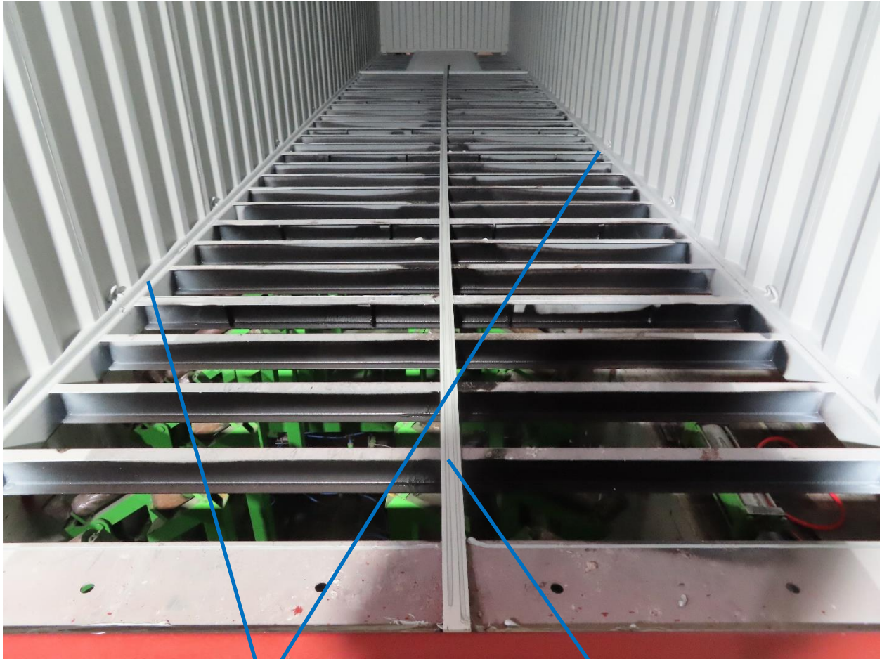
Floor Support Angle FSA
