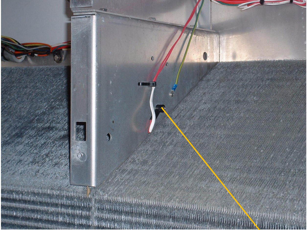
Evaporation coil defrost temperature sensor EVS
